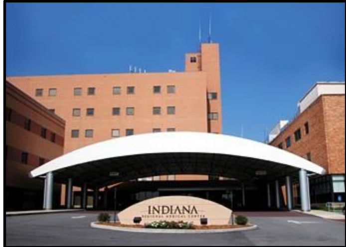
Figure 1 – Current Entrance to IRMC
